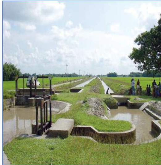
Figure - 4: Cross & head regulators
