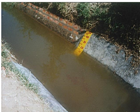
Figure 5 : Canal Gauge
